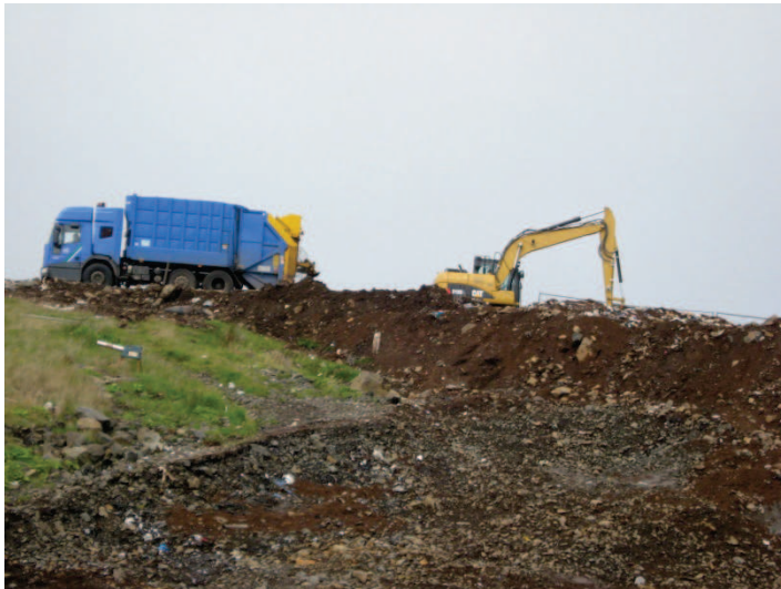
Photograph – Glengorm landfill site, Isle of Mull
